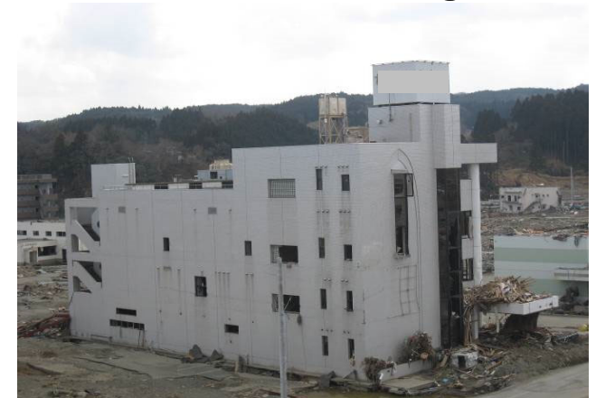
Tsunami evacuation building that withstood tsunami - 200m from the coast - Flood water depth was more than 13m.
